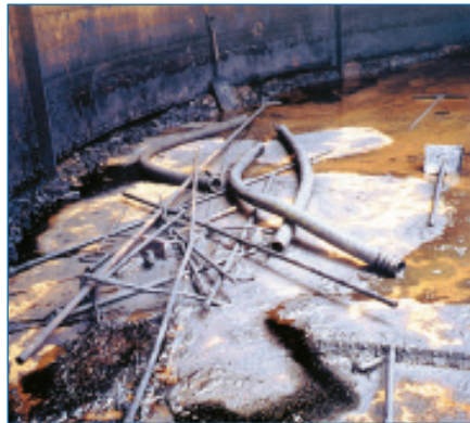
Interior of above-ground gas holder containing residual debris/tar.
